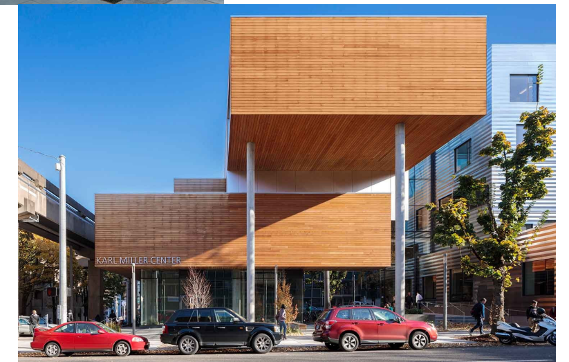
Figure 4-5: Main Entries to building from North/West and South/East show casing entry under program massing
